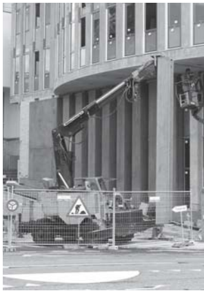
Fig. 39: Top fixing Main support at top of precast element
