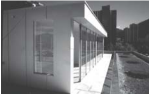
Fig. 11: Bearth & Deplazes: private house "In den Lachen", Chur (CH), 1997
