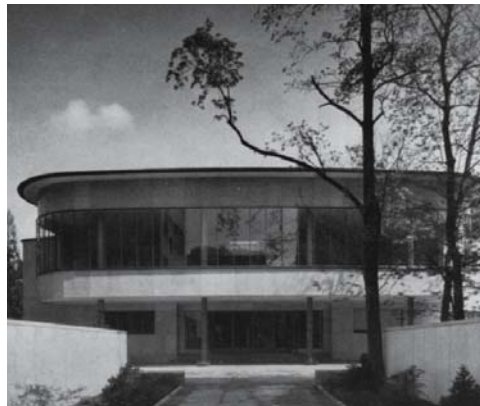
Fig. 40: The dominant horizontal strip window on the upper floor reveals the loadbearing structure.
