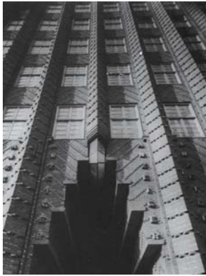
Figure 64: Expressively sculpted facade Fritz Höger: Hannoverscher Anzeiger newspaper building, Hannover (D), 1928
