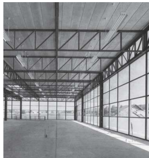
Fig. 16: MAXI building system by Fritz Haller Fritz Haller: USM factory, Münsingen (CH), 1963–84 (extended in four phases)
