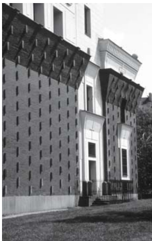
Fig. 3: Lightweight rendered facade over heavyweight masonry Jože Plečnik: Sacred Heart of Jesus Church, Prague (CZ), 1939
