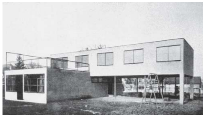
Fig. 114: All traces of the structure are concealed behind masonry panels and render. Artaria & Schmidt: Schaeffer House, Riehen (CH), 1927–28
