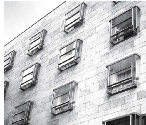
Fig. 34: Cantilevering glass oriels enable good views of the street below. Alejandro de La Sota: Calle Prior apartment block, Salamanca (E), 1963
