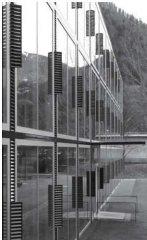
Fig. 248: South facade with entrance External ventilation flaps open
