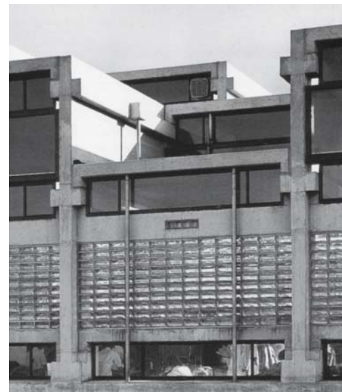
Abb. 58: Use of precast concrete elements and glass Hermann Hertzberger: extension to LinMij plant building, Amsterdam (NL), 1964
