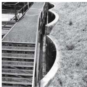
Fig. 28: Retaining wall with “arch” form to resist earth pressure Tank compound, aluminium works, Chippis (CH)
