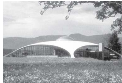
Abb. 70: Shell designed as a fluid form Heinz Isler (with P. Wirz, architect): Kilcher factory, Recherswil (CH), 1965
