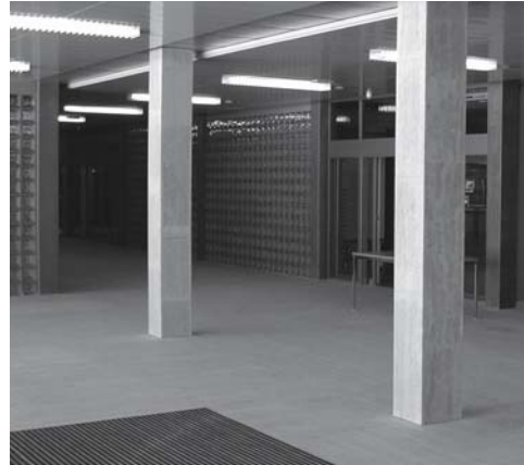
Fig. 235: Entrance area for dining and sports halls The columns in the entrance areas are clad with travertine.
