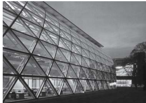
Fig. 74: Glazed barrel-vault roof based on triangular lattice Norman Foster: Faculty of Law, Cambridge (GB), 1995
