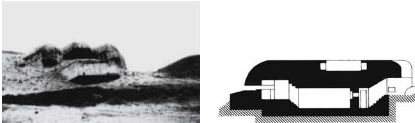
Fig. 51: Bunker in French Atlantic Wall "buried" in the sand (left), longitudinal section (right)
