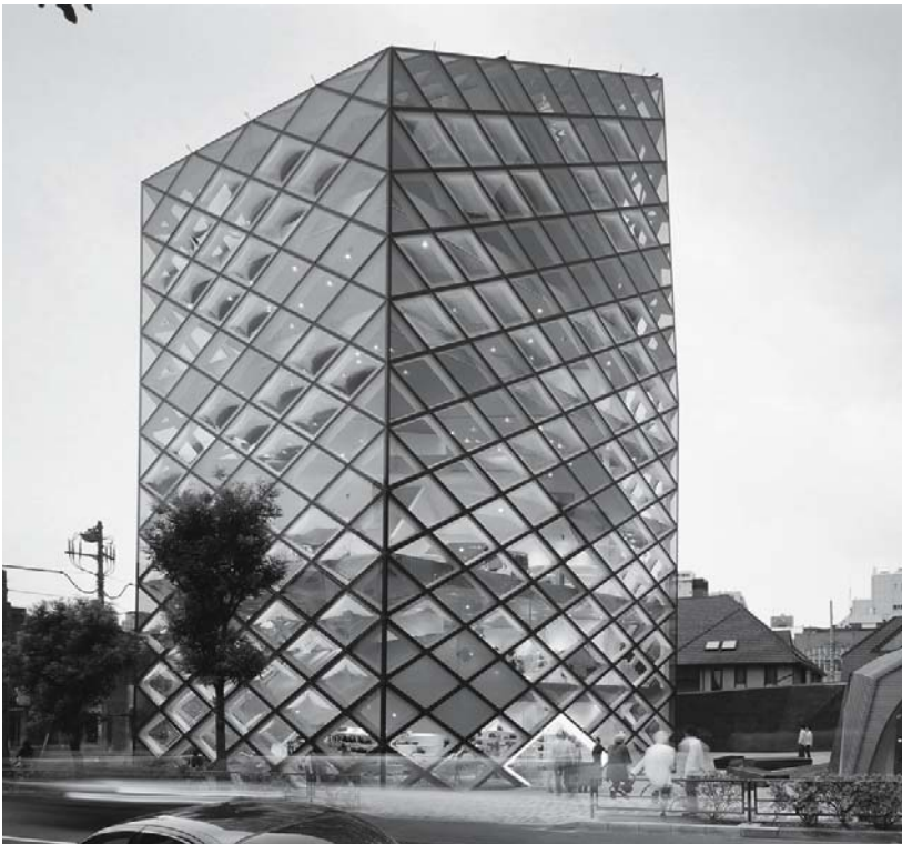
Fig. 19: Loadbearing structure and glazing bars coincide. Herzog & de Meuron: Prada Epicenter Store, Tokyo (J), 2001
