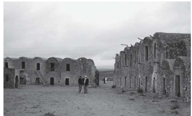
Fig. 56: Inner courtyard View towards the entrance
