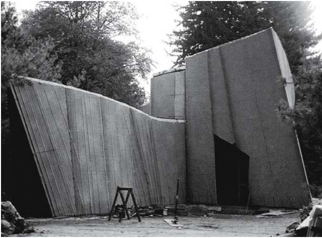
3 Finished assembly of rigid foam panels
