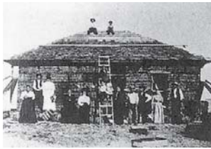
Fig. 6: Built from bales of straw Simonton House in Purdum, Nebraska (USA), 1908
