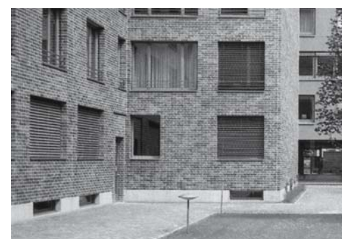
Fig. 59: A raised ground floor leaves room for a basement; natural ventilation and daylight for basement rooms, entrance formed by interruption in plinth Diener & Diener: Wartekhof, Basel (CH), 1993–96
