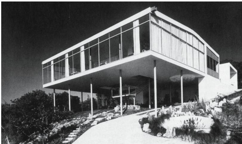
Fig. 116: Transparent, "flying" living room at the front stabilised by compartment-type bedrooms at the rear Lina Bo Bardi: Casa de Vidro, São Paulo (BR), 1951
