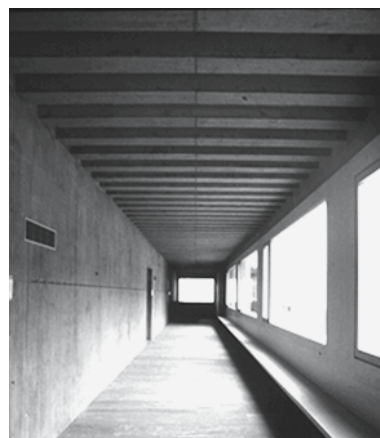
Fig. 4: Bearth & Deplazes: School with hall, Vella (CH), 1997
