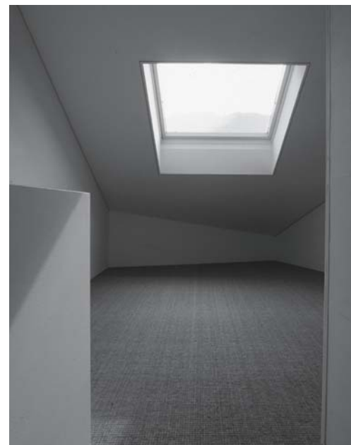
Fig. 306: Window in attic A VELUX roof window used in the traditional way!
