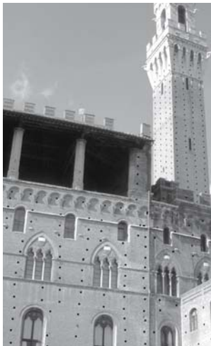
Fig. 15: The pockets for the ends of the scaffold beams are readily visible on the rear of the building.
