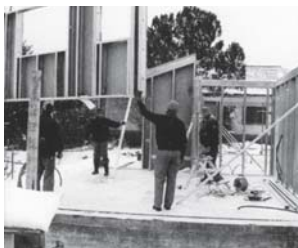
Fig. 7: Erecting a “steel platform frame” The similarity with timber building: sheet metal profiles instead of planks
