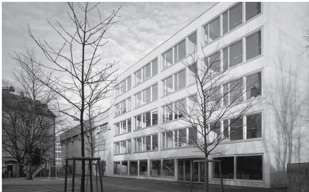
Fig. 153: Entrance elevation fronting the open area
