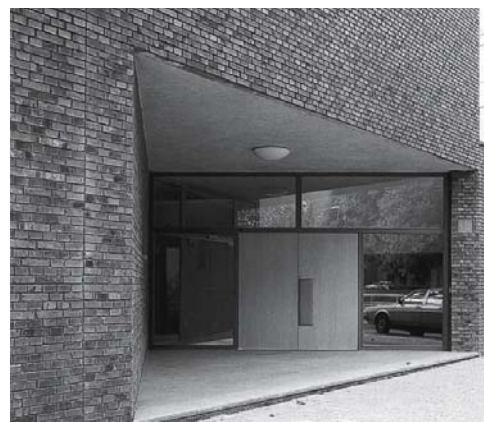
Figure 69: The pattern of English cross bond in double-leaf masonry Hans Kollhoff and Helga Timmermann: Kindergarten, Frankfurt-Ostend (D), 1994
