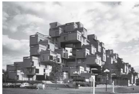
Fig. 133: Stacking of concrete room units (“heavyweight prefabrication”) Moshe Safdie: HABITAT 67, Montreal (CAN), 1966–67
