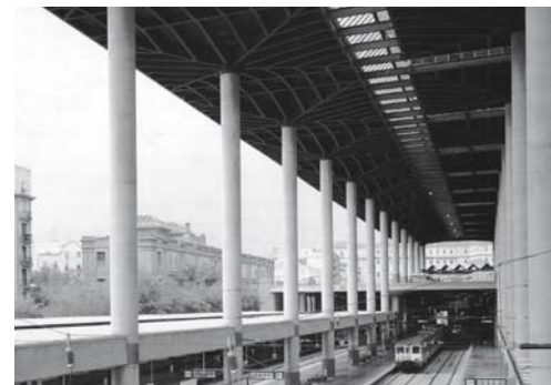
Fig. 80: The structure is legible both internally and externally. Rafael Moneo: Atocha station, Madrid (E), 1984–92
