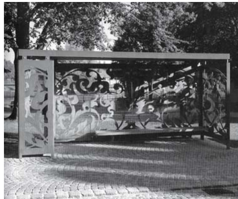
Fig. 52: Bent sheet steel ( d = 12 mm) as a structural element (above); plan, scale approx. 1:140 (left) Hild und K: bus shelter, Landshut (D), 1999
