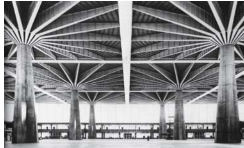
Fig. 76b: Canopies of concrete and steel, bay size 38 x 38 m Pier Luigi Nervi: Hall of Labour, Turin (I), 1961
