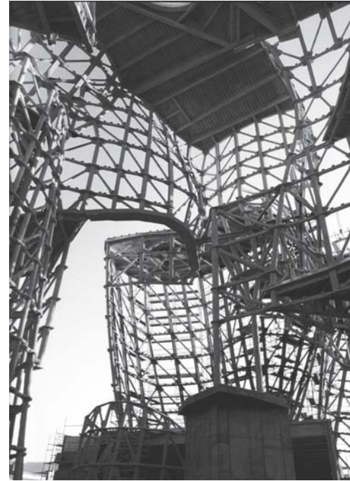
Fig. 18: The dynamic forms were translated into linear lattice structures. Frank O. Gehry: Guggenheim Museum, Bilbao (E), 1997
