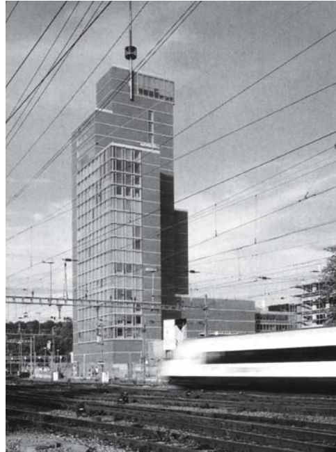
Fig. 58: On the facade the floor slab edges are the only visible part of the loadbearing structure. Burkard, Meyer Architekten: Swisscom headquarters, Winterthur (CH), 1999
