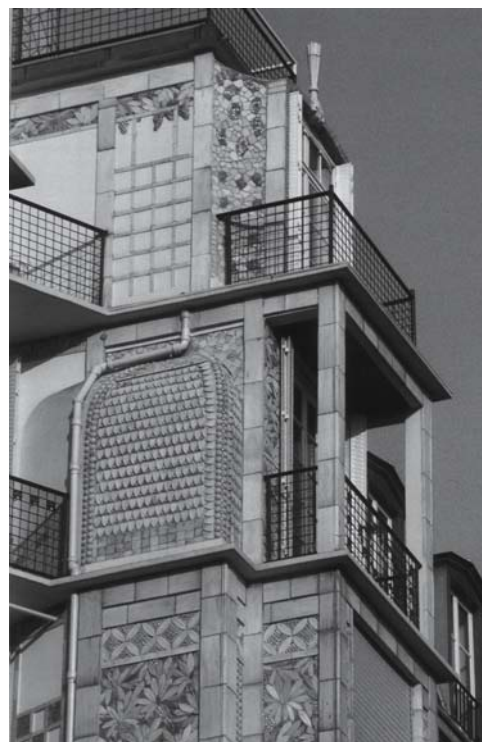
Fig. 5: Playing with variously decorated ceramic panels, view of upper storeys Auguste Perret: apartment block, 25 rue Franklin, Paris (F), 1903–04
