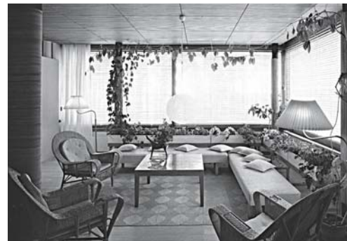
Fig. 88: Internal louvre blinds achieve diffuse interior lighting effects, the surroundings become blurred outlines
