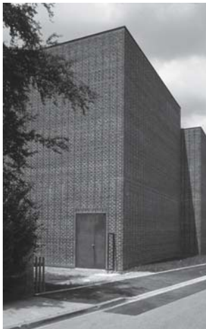
Fig. 65: View from north side
