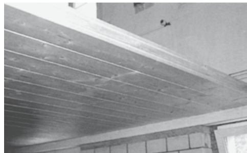
Fig. 8: Staggered positioning of solid timber elements
