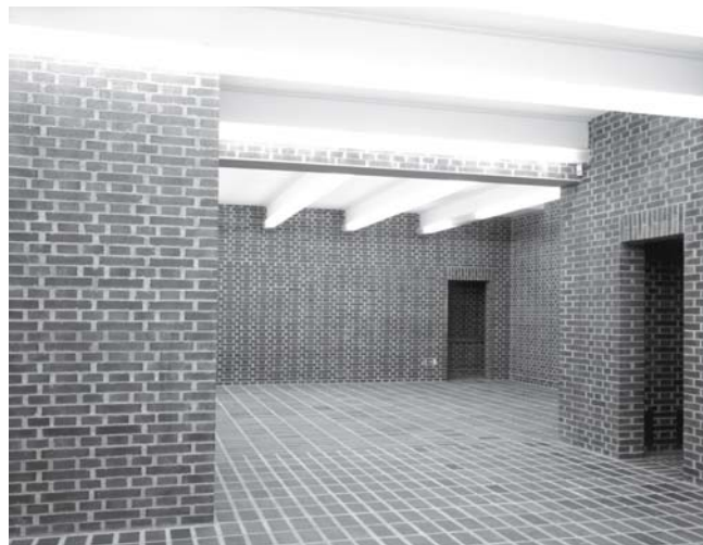
Fig. 83: Artificial lighting fitted to bottom flanges of beams
