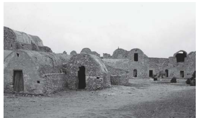
Fig. 57: Inner courtyard Complex at the centre of the ksar
