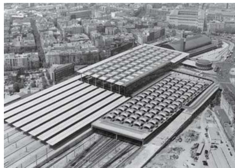
Fig. 78: The table-like construction lends texture to the trainshed roof. Rafael Moneo: Atocha station, Madrid (E), 1984–92
