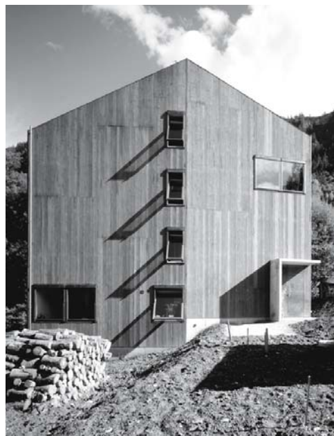
Fig. 303: West facade The linear arrangement of the windows identifies the position of the "static" rooms.
