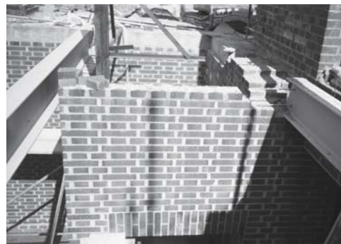
Fig. 75: Bearing for floor beam
