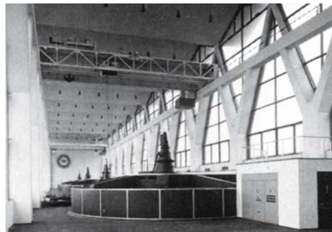
Abb. 68: Folded plate roof supported on Y-columns Hans Hofmann: waterworks, Birsfelden, Basel (CH), 1953/54
