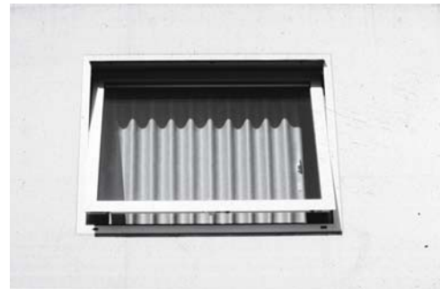
Fig. 121: Horizontal pivot window from outside
