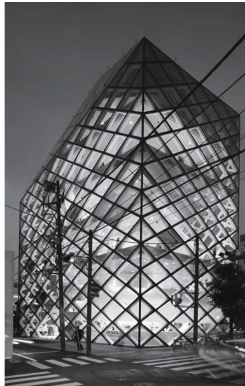
Fig. 20: The rhombuses are bisected at the corners of the building. Herzog & de Meuron: Prada Epicenter Store, Tokyo (J), 2001
