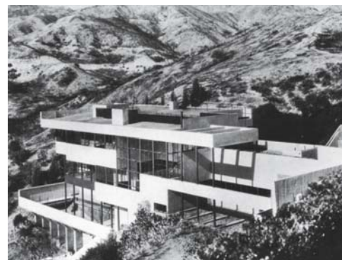
Fig. 8: The steel columns are hardly distinguishable from the window frames. Richard Neutra: Lovell Health House, Los Angeles (USA), 1927–29
