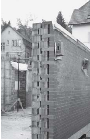
Fig. 48: Ground floor wall at the position of the window flush with the outside face The masonry bond can be clearly seen.
