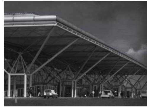
Fig. 79: Modular roof; a second element is suspended between the columns. Norman Foster: Stansted airport, London (GB), 1991
