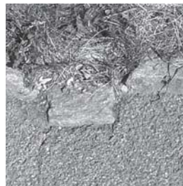
Fig. 38: Boundary stone installed
