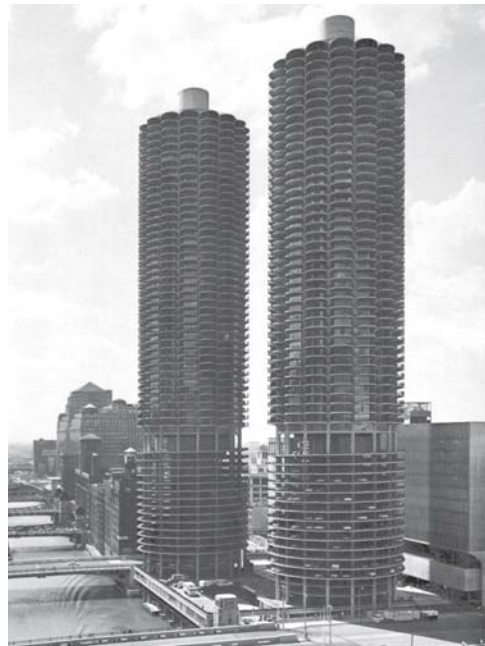
Fig. 11: The cantilevering floor slabs, used as balconies, reinforce the layered nature of the two towers. Bertrand Goldberg: Marina City, Chicago (USA), 1959–64
