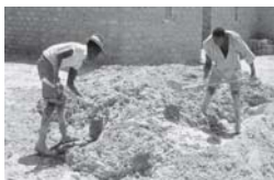
Fig. 2: Earth Mixing with cob and sand
