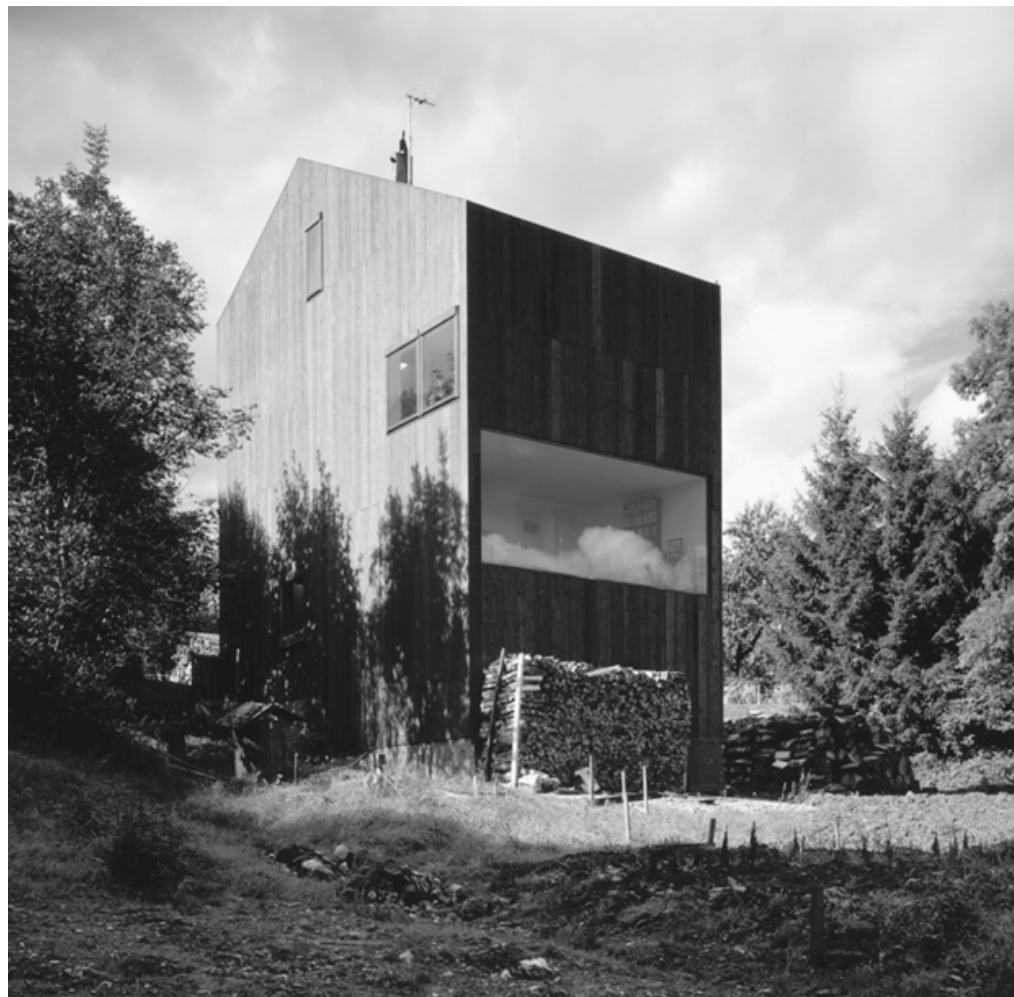
Fig. 286: View from north-east
