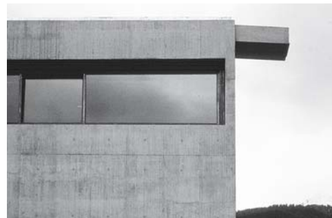
Fig. 149: Inward-opening classroom windows from outside
