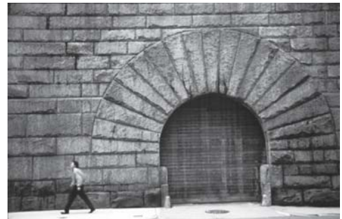
Fig. 18: Rusticated ashlar masonry as a symbol of the power of the state Henry Hobson Richardson: Courthouse and prison, Allegheny County, Pittsburgh (USA), 1888
