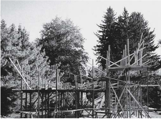
1 Horizontal wooden templates positioned and fixed with the help of a scaffold
