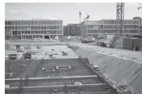
Fig. 43: Sloping sides stabilised with plastic film
