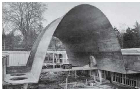
Abb. 69: Shell designed with perfect form (parabola), shell thickness approx. 6 cm. Robert Maillart: Cement Industry Pavilion for Swiss National Exhibition, 1939
