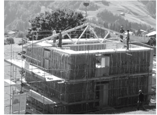
4 Structural shell almost complete, only the protective layer of render has yet to be applied
