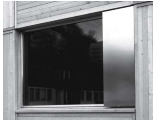
Fig. 281: Sunshading Sunshading in the form of an aluminium shutter in front of the ventilation light plus a fabric awning in front of the fixed light
