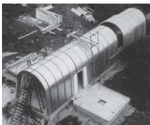
Fig. 54: Loadbearing structure and building envelope united in the form of semicircular, loadbearing sandwich elements, shown here almost complete. Jean Prouvé: La Méridienne de l'observatoire, Paris (F), 1951
