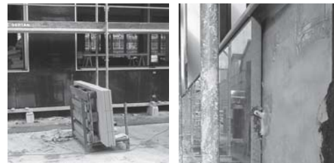
Fig. 49: Stone facade Fixed with cast-in dowels
