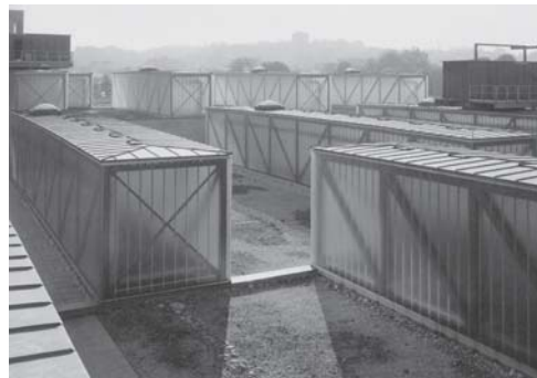
Fig. 62: The lantern lights (clad with patterned glass) span from wall to wall. Herzog & de Meuron: locomotive depot “Auf dem Wolf”, Basel (CH), 1995
