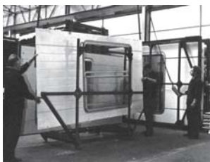
Fig. 14: Industrial manufacture of facade elements: single element Jean Prouvé: CIMT, Paris (F), c. 1955
