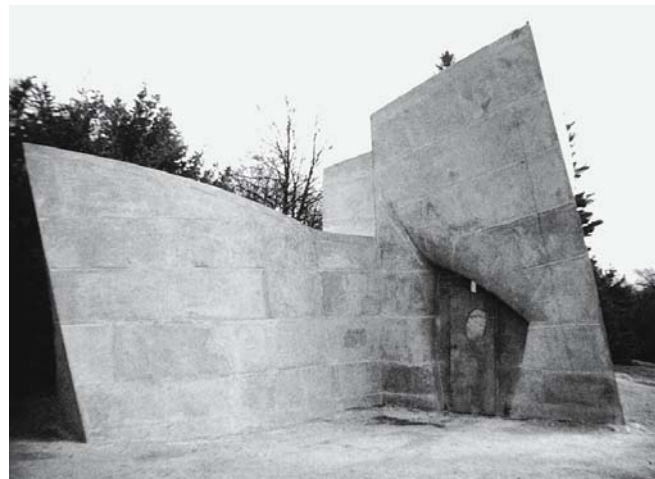
6 Gate House cleaned and prepared ready for painting
