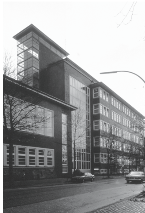
Fig. 20: Example of a modern building using facing masonry Fritz Schumacher: Wendenstrasse School, Hamburg-Hammerbrook (D), 1929
