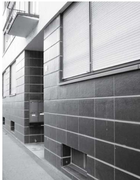
Fig. 67: Painted concrete and ceramic tiles as protection against weather and soiling, and also providing a figurative plinth function Otto Rudolf Salvisberg: apartment block, Zurich (CH), 1936
