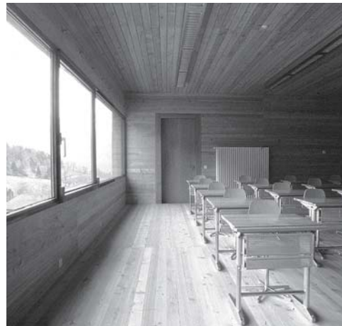
Fig. 148: Inward-opening classroom windows from inside
