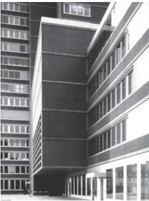
Fig. 78: Facade assembled from three different prefabricated elements Burkard Meyer Partner: Swisscom headquarters, Winterthur (CH), 1999
