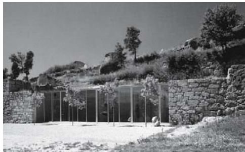
Fig. 18: Interlacing of building and topography with (retaining) walls Eduardo Souto de Moura: Baiao House, Baiao (P), 1991–93
