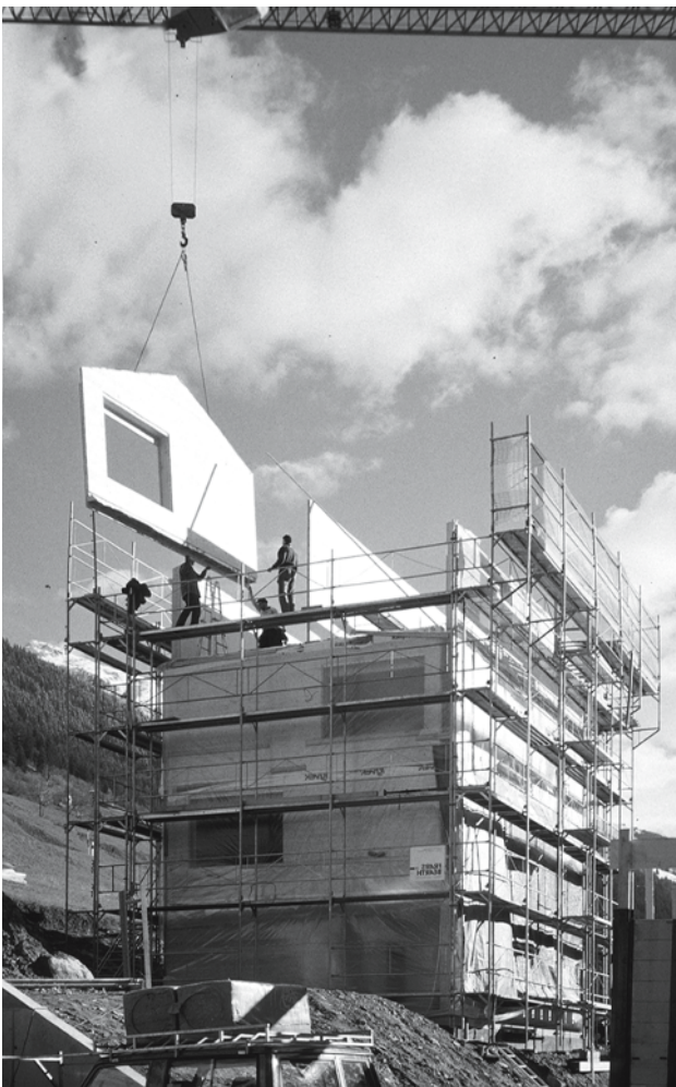
Figs 1 and 2: Solid timber panel construction, completed with shingle cladding (top); erecting the panels (bottom)
