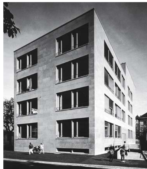
Fig. 2: Steel frame concealed behind brick facade Diener & Diener: Vogesen School, Basel (CH), 1994
