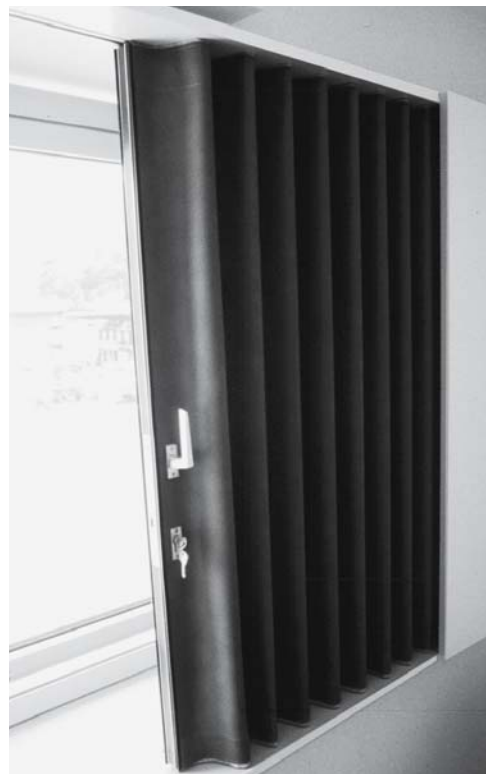
Fig. 112: Window with “imitation leather bellows”
