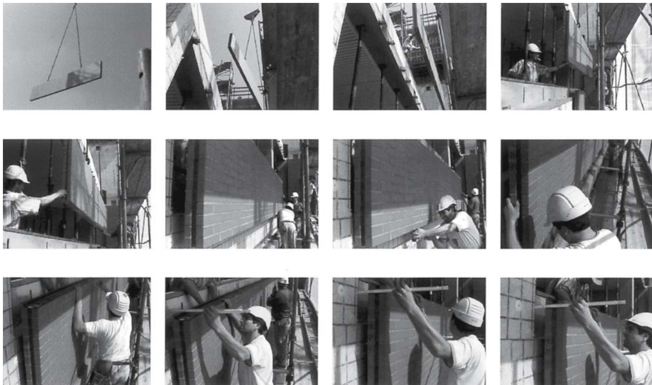
Fig. 77: Examples from a Swiss manufacturer: "preton" element catalogue Masonry elements being erected at the Swisscom headquarters by Burkard, Meyer in Winterthur
