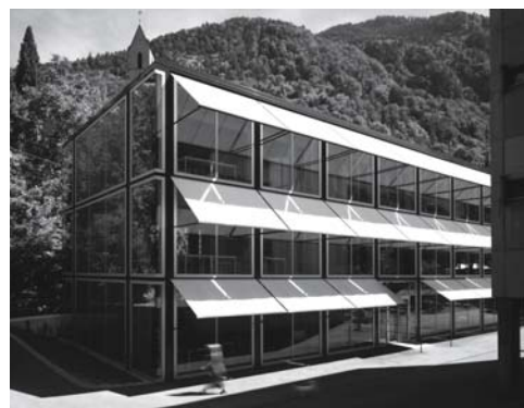
Fig. 253: South facade with awnings extended The facade is given relief; the omission of one awning marks the entrance (fixed canopy).
