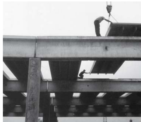
Abb. 52: Precast concrete beams in a framed building Angelo Mangiarotti: industrial building, Bussolengo (Brescia), 1982
