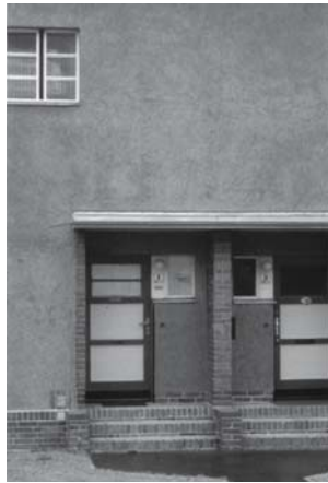
Fig. 50: Bold colours distinguish the entrance and so the door is singled out as a key design element
