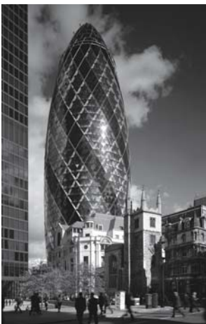
Fig. 21: The size of the rhombuses matches the form of the building. Foster & Partners, Swiss Re Tower, London (GB), 2000–04
