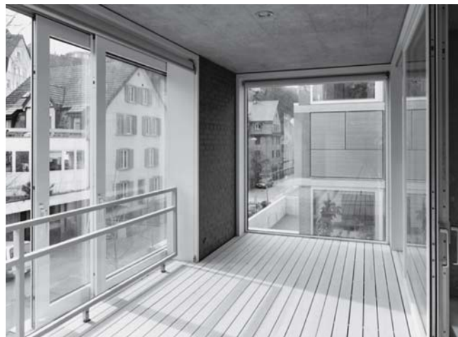
Fig. 62: Veranda Unheated intermediate zone acts as extension to living room and also as balcony.
