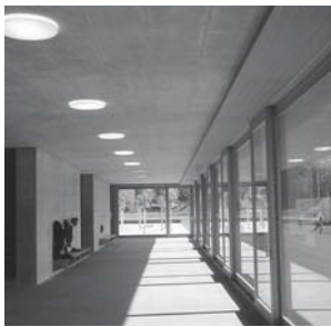
Fig. 31: Insulation to the soffit along the perimeter concealed behind timber cladding Bünzli & Courvoisier: Linde school, Niederhasli (CH), 2003
