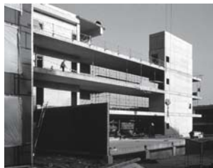
Fig. 267: Concrete cores Under construction, 1997; the concrete floors support only their own self-weight and therefore large spans and cantilevers are possible.
