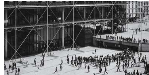
Fig. 8: A ramp links the underground entrance with the surrounding street level. Renzo Piano, Richard Rogers: Centre Pompidou, Paris (F), 1977
