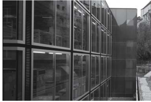
Fig. 243: North facade Staircase tower bracing the whole structure; frameless glass curtain wall
