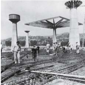
Fig. 76a: Canopies under construction Pier Luigi Nervi: Hall of Labour, Turin (I), 1961
