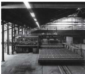
Fig. 29: Clay brick production "Green bricks" on traversers prior to drying and firing
