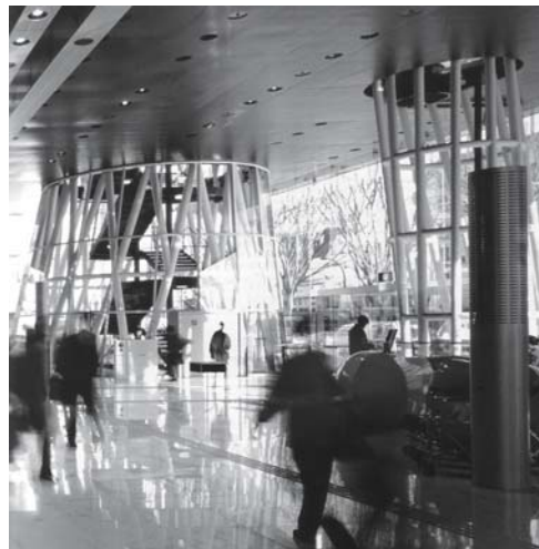
Fig. 72b: The corner columns house the stairs. Toyo Ito: Mediothek, Sendai (J), 2001
