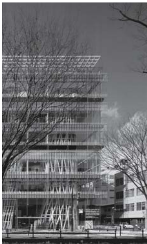
Fig. 72a: The four corner columns with intersecting linear members function in a similar way to Suchov's mast. Toyo Ito: Mediothek, Sendai (J), 2001
