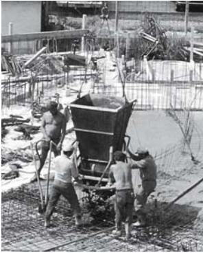
Fig. 21: Placing concrete by crane skip
