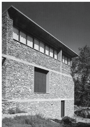
Fig. 38: The horizontal strip window separates the roof from the solid walls. Herzog & de Meuron: House in Tavole (I), 1988
