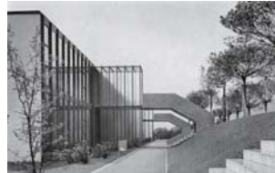
Fig. 13: Spoil used to form an embankment, as noise barrier and to provide access to upper floor Fritz Haller: Bellach School, Solothurn (CH), 1959
