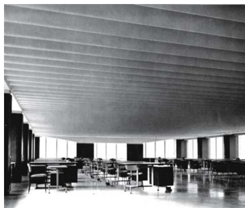
Fig. 9: Galbani office building Milan (I), 1955/56 Reinforced concrete floor by Pier Luigi Nervi Design: E. Soncini, A. Pestalozzo
