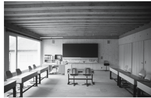
Fig. 23: Classroom with ribbed concrete soffit
