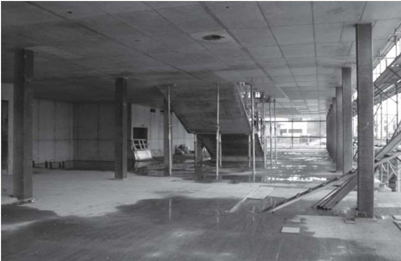
Fig. 215: View during construction Entrance hall to secondary school, floor slab over ground floor and precast concrete columns
