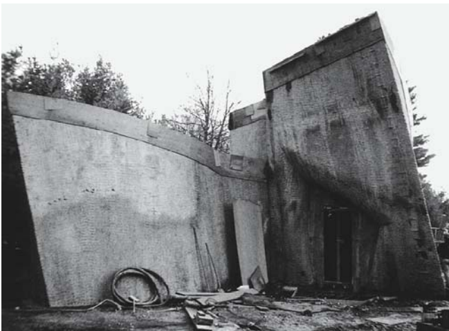
5 Building coated with the first layer of sprayed concrete
