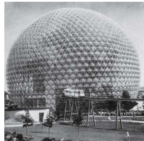
Fig. 71: The truncated sphere has a base diameter of 110 m. Buckminster Fuller: USA Pavilion, EXPO 67, Montreal (CAN), 1967
