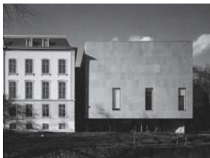
Fig. 42: Tall windows create a link between old and new building. Diener + Diener: Pasquart Centre, Biel (CH), 1999
