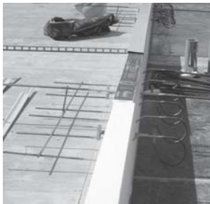
Fig. 33: Example of insulated reinforcement being installed
