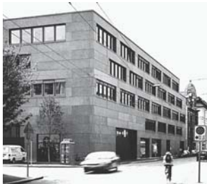
Fig. 7: Diener & Diener: Warteckhof mixed residential and commercial development, Basel (CH), 1996
