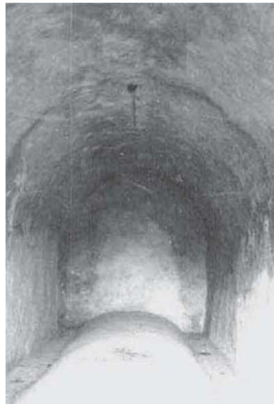
Fig. 67: Ghorfa Interior view, upper floor, with vaulted floor
