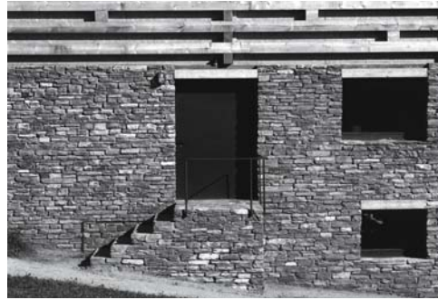
Fig. 65: The difference in height on existing terrain is accommodated within the solid plinth for the timber structure above. Gion Caminada: factory, Vrin (CH), 1999
