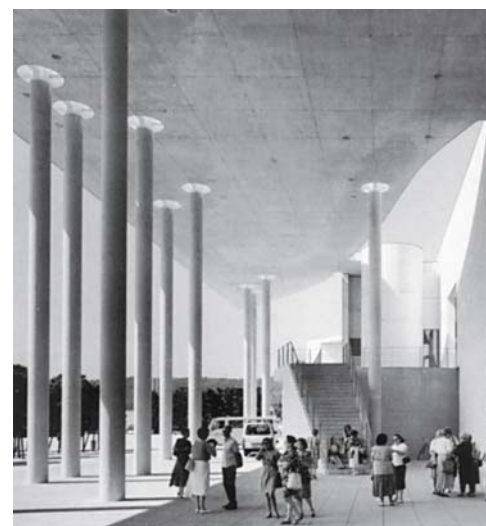
Abb. 54: Spun-concrete columns, connected to reinforced concrete roof via steel web plates. Axel Schultes: art gallery, Bonn (D), 1992
