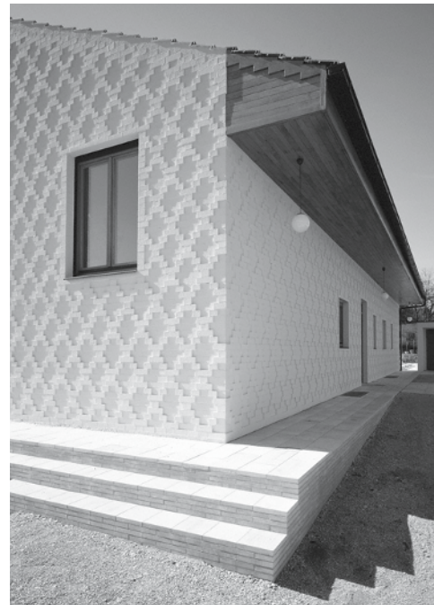
Figure 63: Ornamentation through relief (bricks offset within depth of wall) Hild & K: Wolf House, Aggstall (D), 2000
