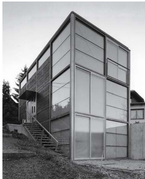
Fig. 59: The square grid visible on the facade is only a covering to the load-bearing elements behind. Georg Marterer: teahouse in Neustift am Walde, Vienna (A), 1998
