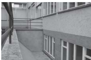
Fig. 60: Lightwell with fully habitable basement rooms Steger & Egender: Art School, Zurich (CH), 1933
