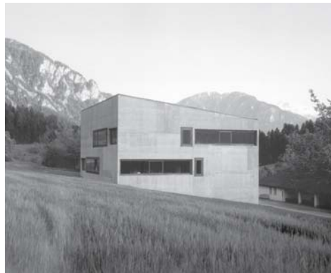
Fig. 64: A building growing monolithically out of the hillside Valerio Olgiati: school, Paspels (CH), 1998
