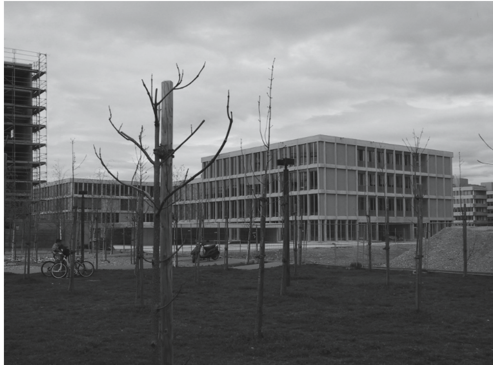
Fig. 199: General view of school buildings
