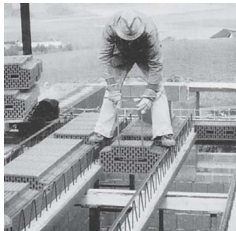
Fig. 2: Fitting the individual Hourdis-type elements between the reinforced concrete beams
