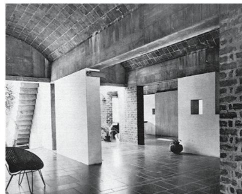
Fig. 72: Box frames as a governing design principle Le Corbusier: private house (Sarabhai), Ahmedabad (India), 1955
