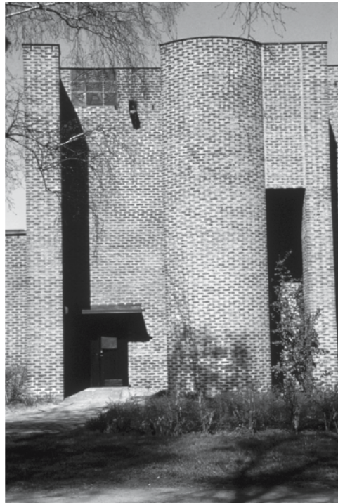
Fig. 10: Bed joint widths approaching the height of an individual brick Sigurd Lewerentz: Markus Church, Björkhagen near Stockholm (S), 1960
